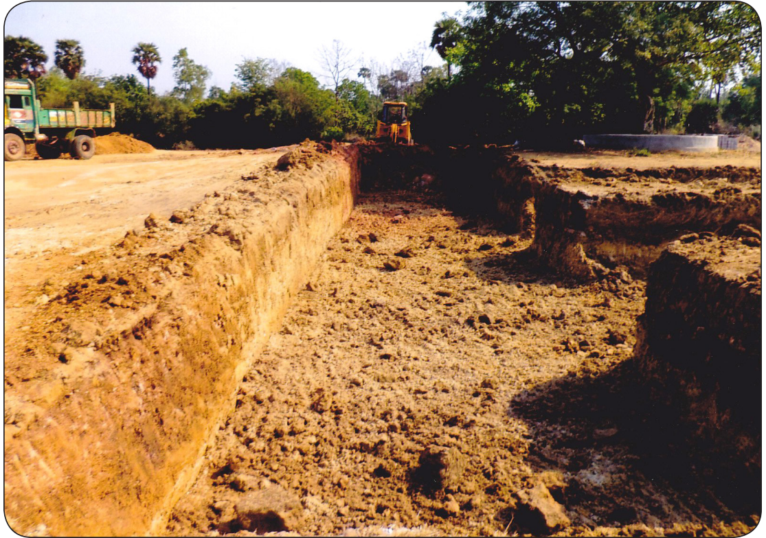
The foundation for the vocational school is being dug.
