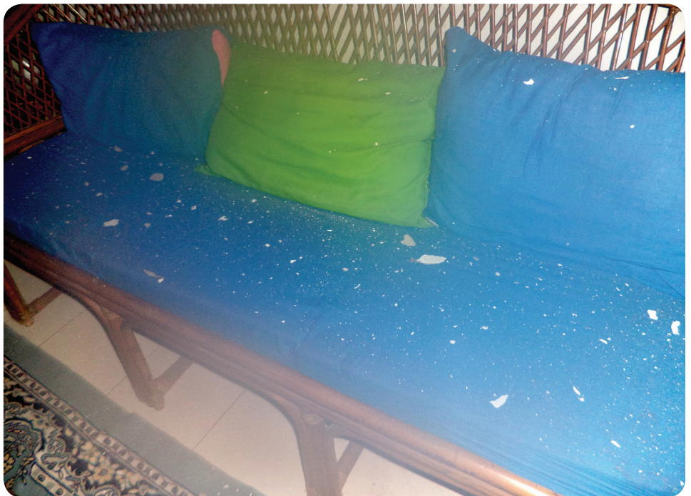
Top photo: The hole in Darlene's wall from the lightning strike. Photo above: The pieces of plaster on her couch.
