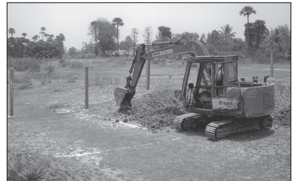
Construction begins on the new campus
