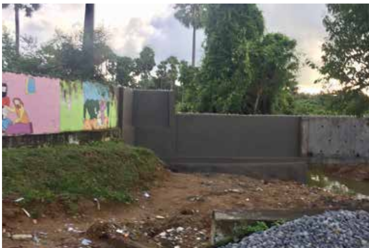
Pictured above: reconstruction of the wall that Cyclone Gulab took out complete with a new system for mitigating flood waters.
