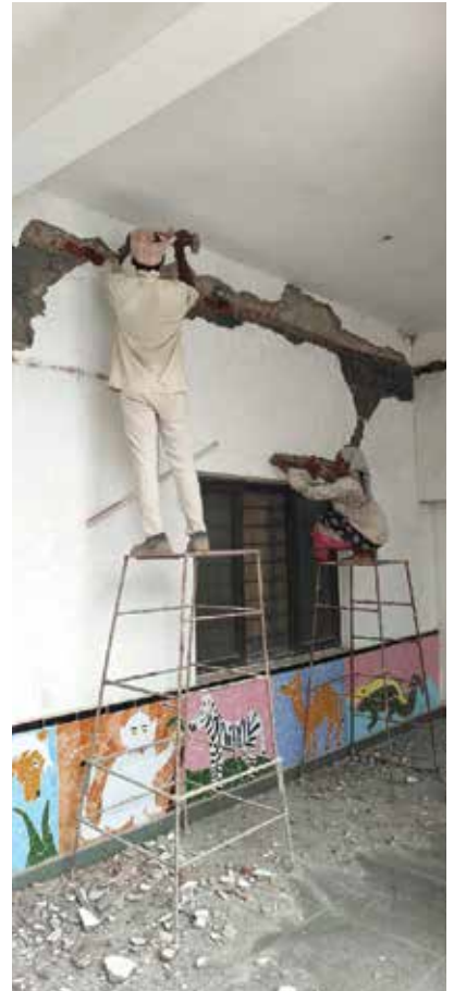
Mason using mallet and chisel to remove water-damaged concrete from wall.
